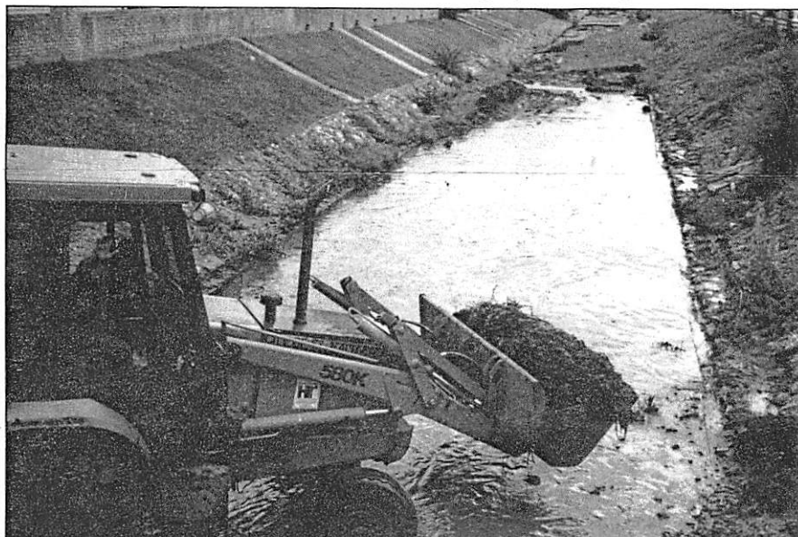
A Construction Department crew recently plowed into Weicher Creek near Dutchmans Lane, dredging silt from the creekbed.
