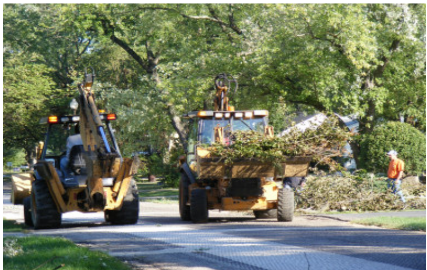
City crews wasted no time re-opening streets and carting away debris.
