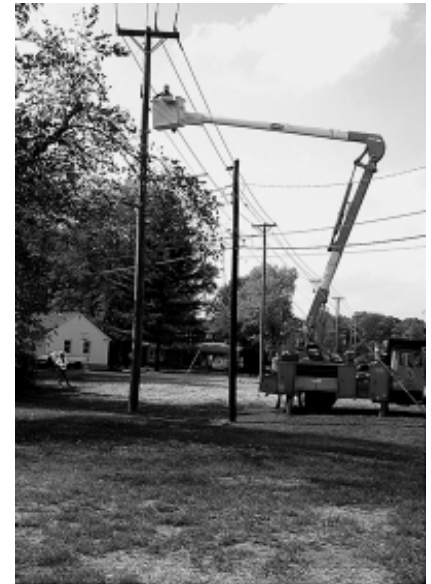
The Westport Road widening project is moving east toward St. Matthews; this crew was stringing cable on a recent sunny day.
