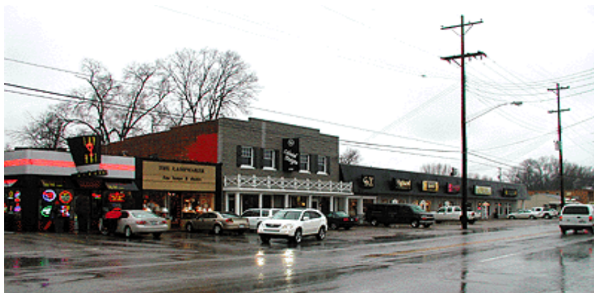
The south side of Lexington Road also has been spruced up, and is busier than ever.
