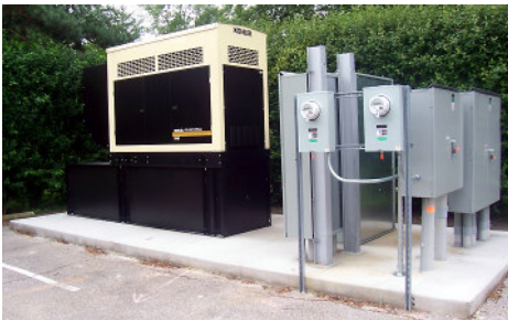
First and last chance to see the city's sleek new emergency generator: It's now hidden by an eight-foot fence.
